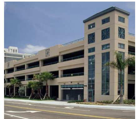
Judicial Center Parking Garage, PBC
