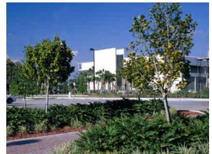
North County Government Complex, PBG
